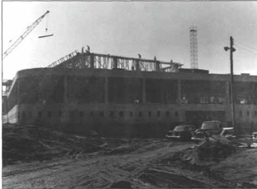
Original Headquarters Building under construction, 1950-60
