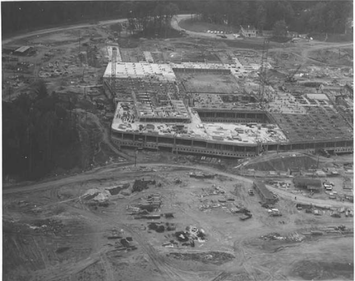
The state of construction in October 1959.
